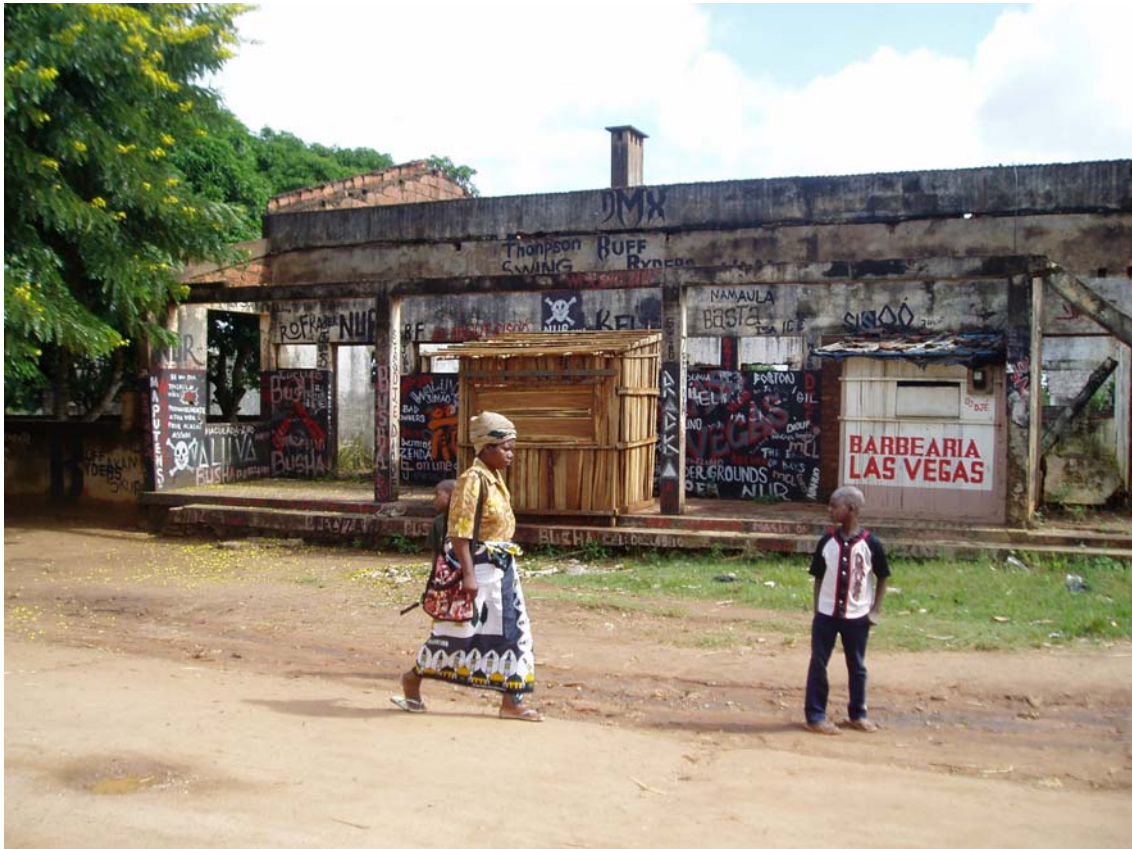
A ruined building in the town of Morrumbala.
